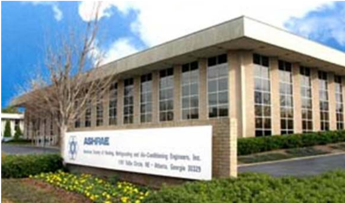
Figure F.1 The ASHRAE Headquarters Building (Photograph Courtesy of ASHRAE).
